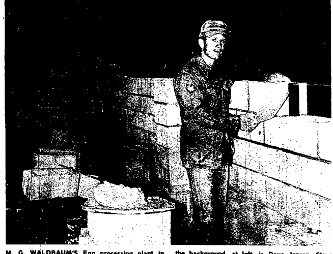
M. G. WALDBAUM'S Egg processing plant in Wakefield will soon have a new building measuring 140 feet long and 60 feet wide, to be used for a truck garage, and will also contain compressors for freezer units in nearby buildings. In the background, at left, is Dave Jensen. Steve VonMinden, Ponca, finishes laying a block in the right foreground. Both are employees of Book Construction Co., Ponca.
